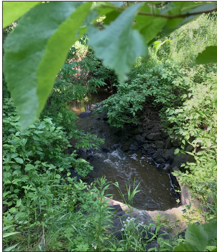
The 1970s structure forced the 20-foot-wide stream through a 4-foot pipe, seen here in 2017. Photo Credit: Ann Wessel, BWSR
